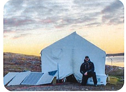
Off-grid solar system, Nunavut
